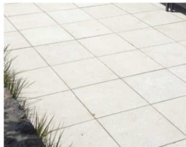
Broom finished Concrete Pedestrian Paths
